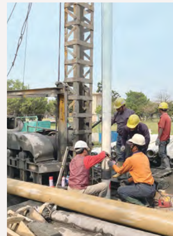
鑿井工程 Well drilling engineering
