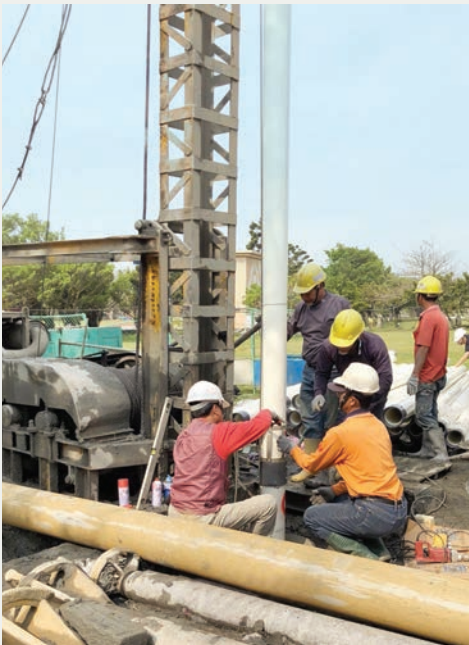
鑿井工程 Well drilling engineering
